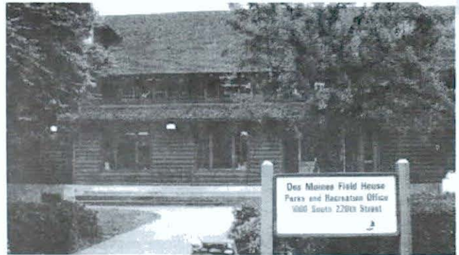
The Field House received a fresh exterior coat of paint.
