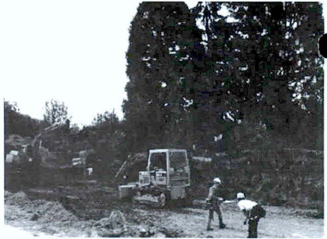
A rockery is being built around the root system of giant trees.
